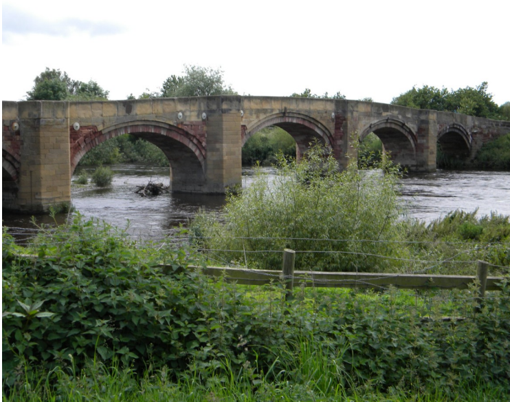
Old Bridge at Bangor on Dee
